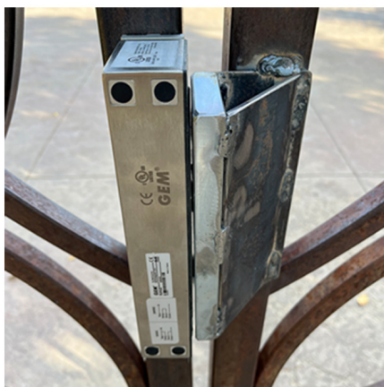
The crew from England Fence installed a new latch on the main entrance gate to the Gardens in October. The new device has a programmable, magnetic locking mechanism.
